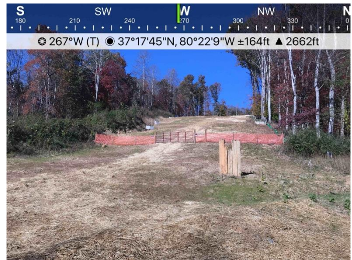
Figure 4: Area near MLV 26 is stabilized and ESC's are in place.
