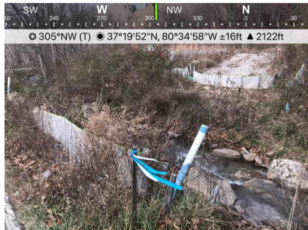
Figure 8: Designated crossing S-Y2. ECD's are in place.
