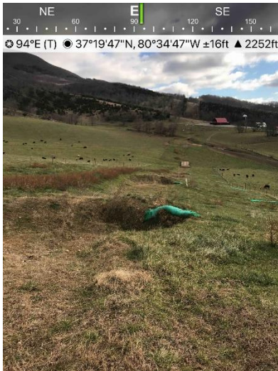
Figure 7: Looking from St 10941+20 toward 10948+50, area is stabilized.
