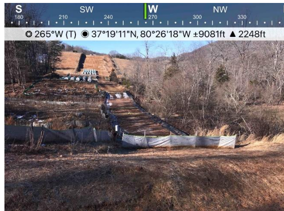
Figure 4: Designated stream S-0013, ECD's are in place.
