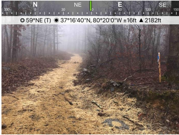
Figure 1: AR –MN266 has been stabilized with mulch.
