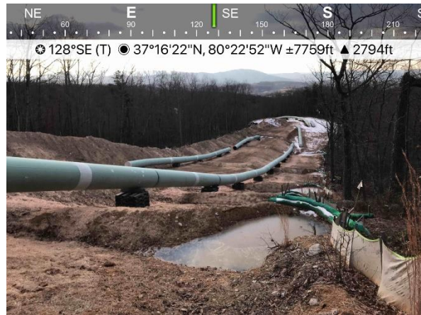
Figure 2: St11677+00 ECD's are installed and the area is temporarily stabilized.
