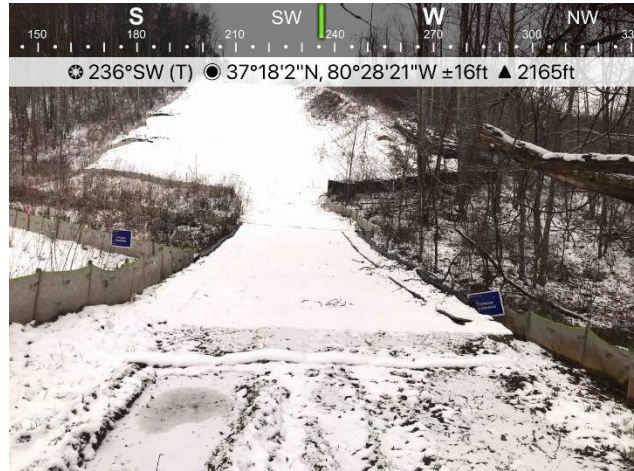
Figure 4: Designated crossing S-NN12 ECD's are in place.
