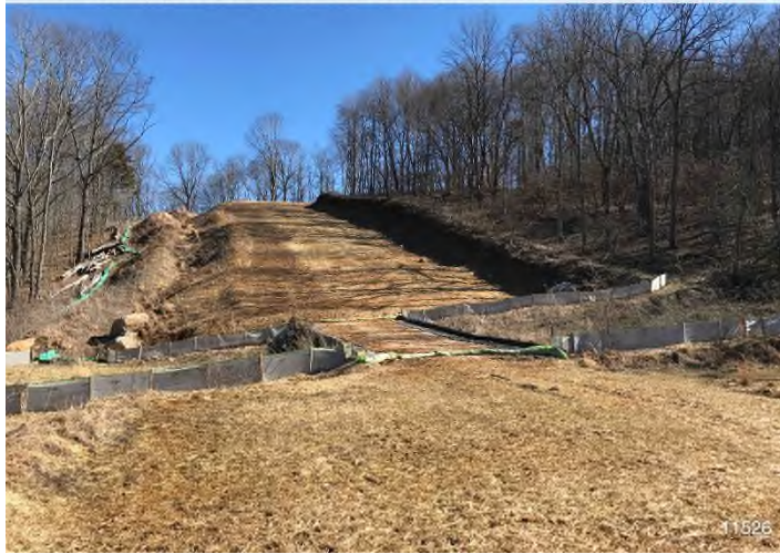
Figure 3: STA 11526+00 – Controls in place and functioning properly. Area stabilized with straw.
