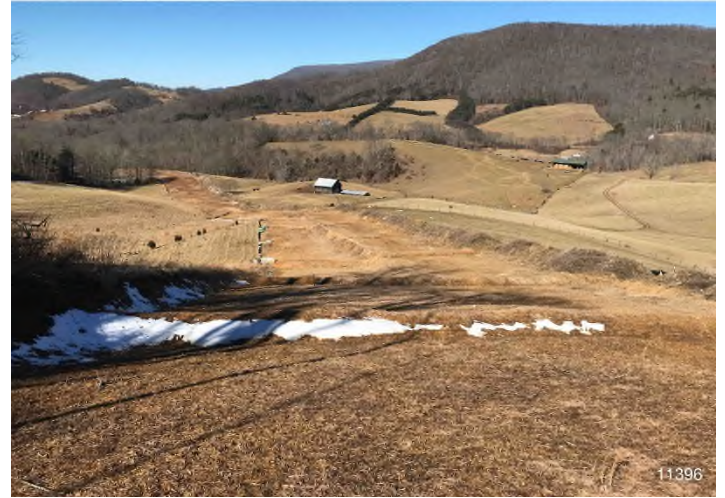
Figure 4: STA 11494+00 – Controls in place and functioning properly. Area stabilized with straw.
