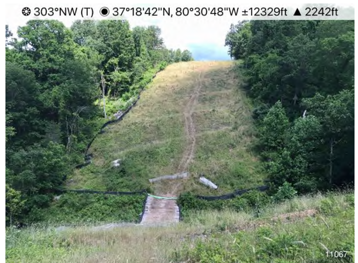
Figure 4: STA 11067+00 – Controls in place and functioning properly. Area stabilized.
