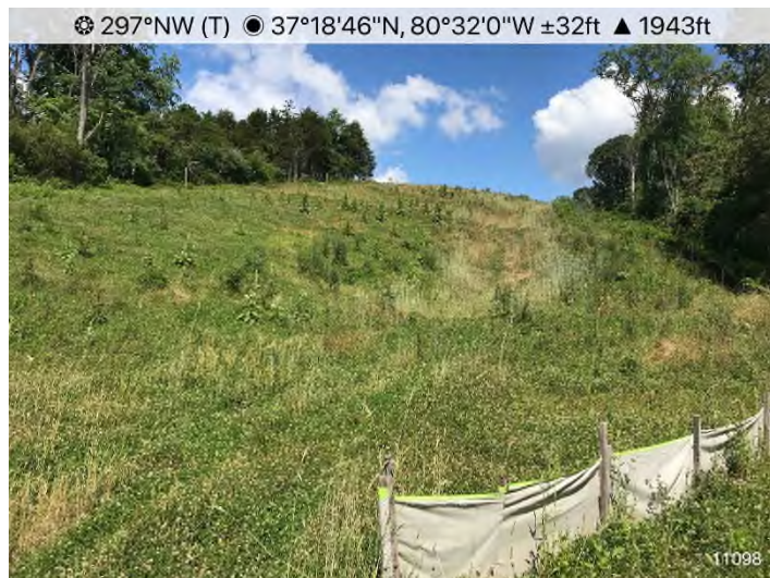
Figure 3: STA 11098+00 – Controls in place and functioning properly. Area stabilized.
