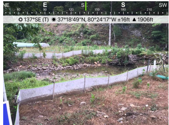
Figure 4: Designated crossing S-006, ECD's in place and effective.
