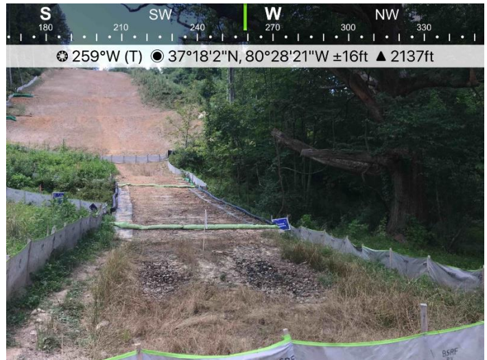
- Figure 4: Designated stream S-NN12, ECD's are in place.
