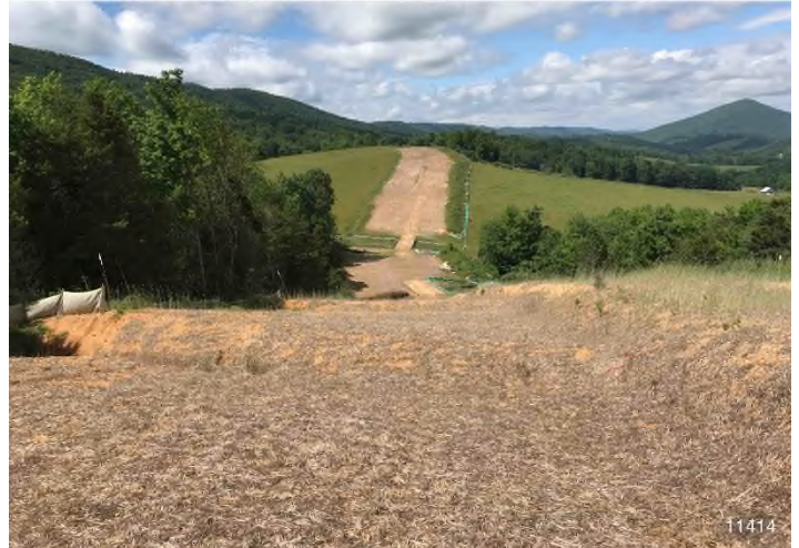
Figure 4: STA 11414+00 – Controls in place and functioning properly. Area stabilized with straw.
