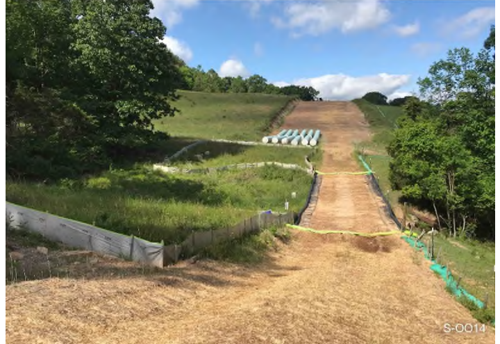
Figure 4: STA 11414+00 – Controls in place and functioning properly. Area stabilized with straw.
