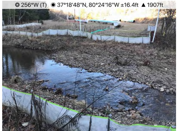
Fig. 4: STA 11231+00 – Controls in place and functioning properly. Area stabilized with straw and vegetation.
