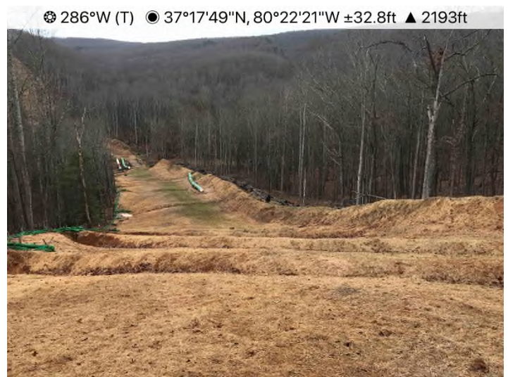
Fig. 4: STA 11755+00 – Controls in place and functioning properly. Areas stabilized with straw.
