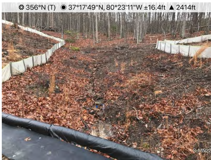
Fig. 3: Stream S-MN22 – Controls in place and functioning properly.
