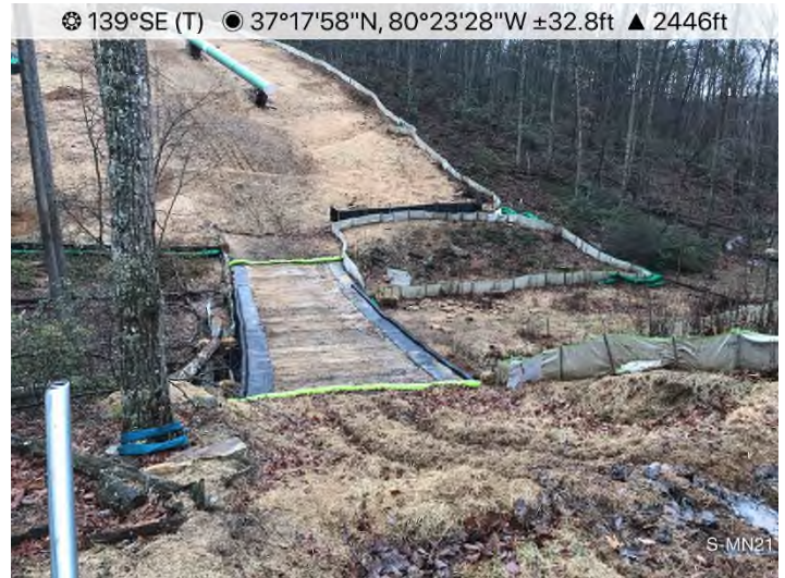
Fig. 4: STA 11755+00 – Controls in place and functioning properly. Areas stabilized with straw.
