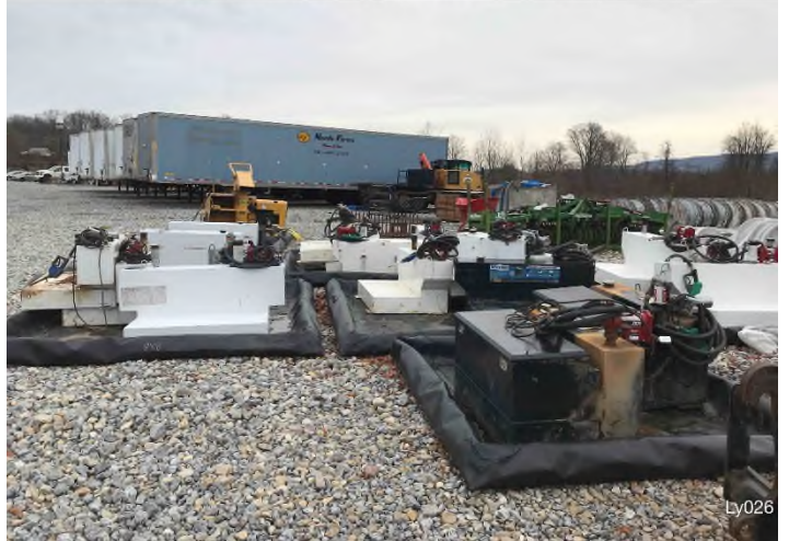
Fig. 4: Laydown Yard 028 – Secondary containment placed under equipment storage to contain potential leaks.
