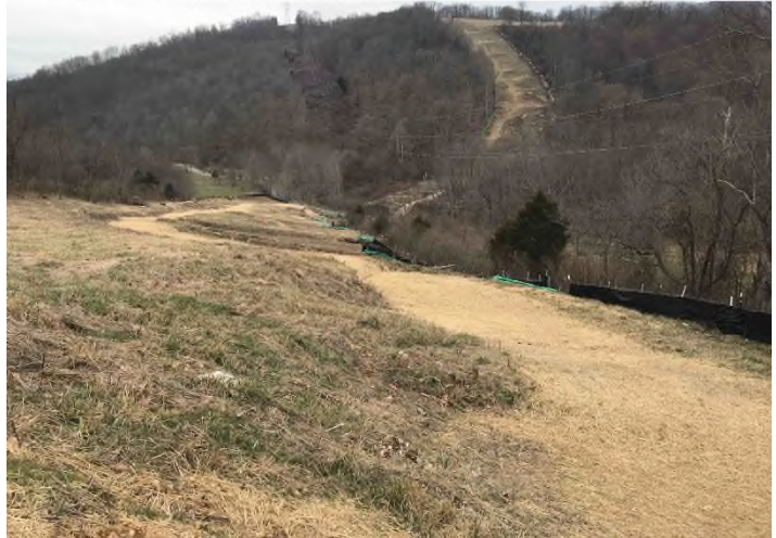
Figure 4: STA 10932+00 – Controls in place and functioning properly. Area stabilized with straw.
