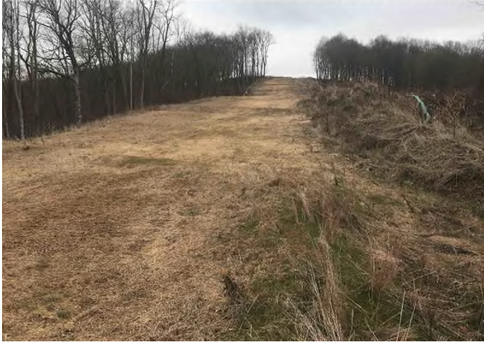
Figure 3: STA 10970+00 – Controls in place and functioning properly. Area with straw.
