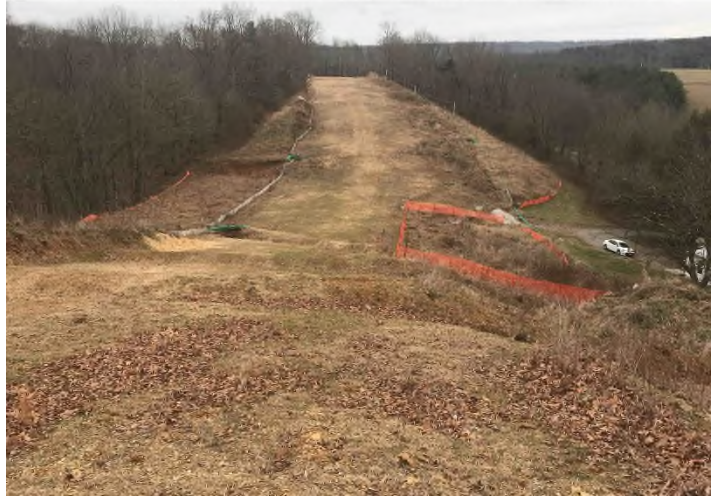
Figure 4: STA 10932+00 – Controls in place and functioning properly. Area stabilized with straw.
