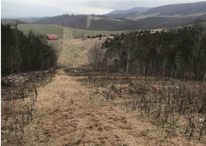
Figure 3: STA 10970+00 – Controls in place and functioning properly. Area with straw.
