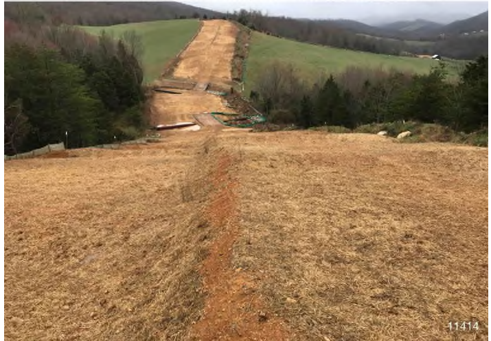
Figure 8: STA 11414+00 – Controls in place and functioning properly. Area stabilized with straw. No erosion evident.
