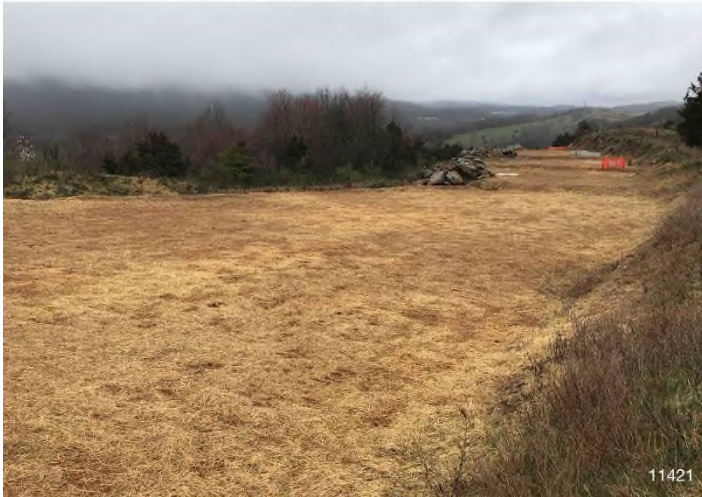
Figure 7: STA 11421+00 – Controls in place and functioning properly. Area stabilized with straw. No erosion evident.
