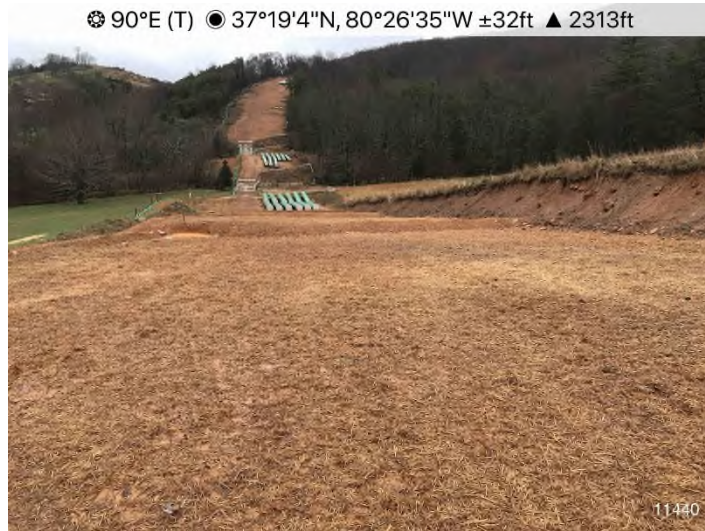
Figure 3: STA 11440+00 – Controls in place and functioning properly. Area stabilized with straw. No erosion evident.
