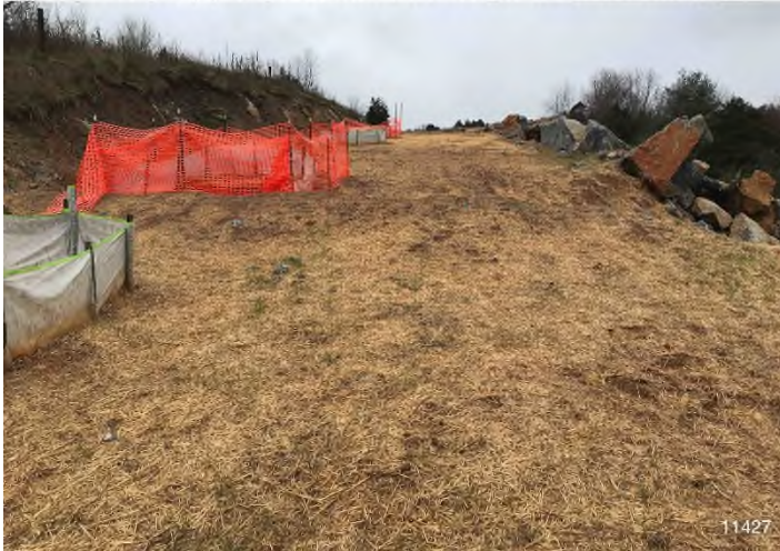
Figure 7: STA 11421+00 – Controls in place and functioning properly. Area stabilized with straw. No erosion evident.
