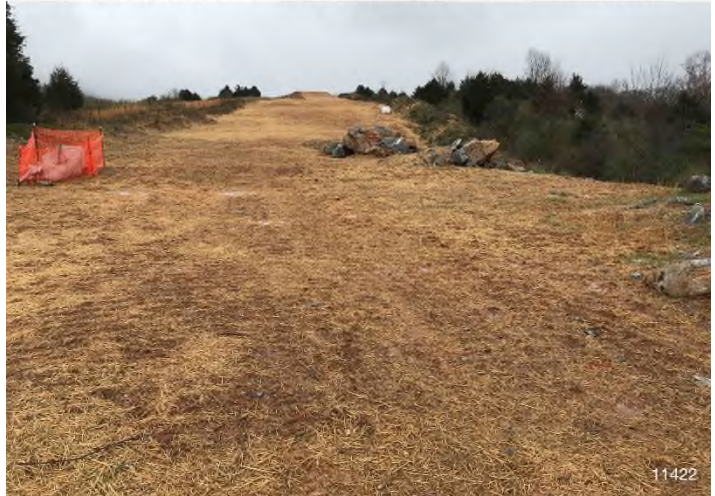
Figure 8: STA 11414+00 – Controls in place and functioning properly. Area stabilized with straw. No erosion evident.
