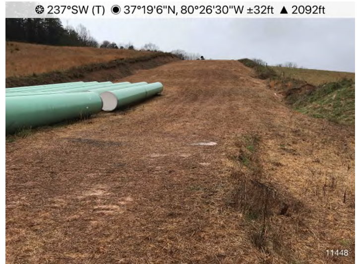
Figure 4: STA 11439+00 – Controls in place and functioning properly. Area stabilized with straw. No erosion evident.
