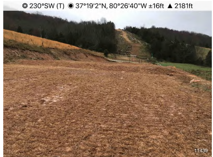
Figure 4: STA 11439+00 – Controls in place and functioning properly. Area stabilized with straw. No erosion evident.
