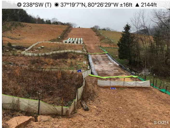
Figure 3: STA 11440+00 – Controls in place and functioning properly. Area stabilized with straw. No erosion evident.
