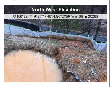
Figure 3: Designated crossing S-IJ52, ECD's are in place
