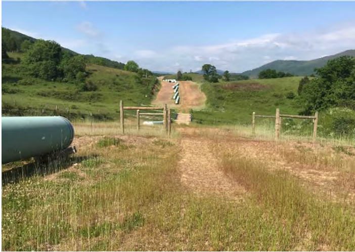
Figure 3: STA 11616+00 – Controls in place and functioning properly. Area stabilized with straw.
