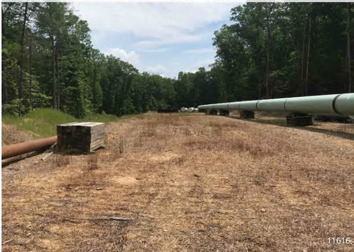
Figure 3: STA 11616+00 – Controls in place and functioning properly. Area stabilized with straw.
