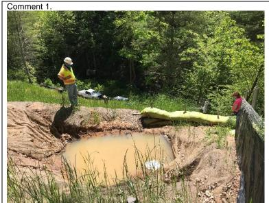
Eroded waterbar will overflow over dike.
