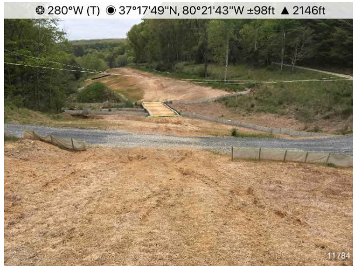
Figure 3: Stream S-RR13 – Controls in place and functioning properly along S-RR13.
