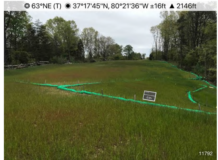
Figure 4: STA 11608+40 – Controls in place and functioning properly along Craig Creek.
