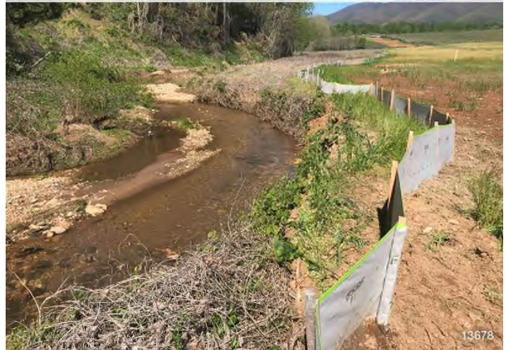
Figure 4: STA 13678+00 – Recent P1 repair along Teels Creek (S-E28). Note incised stream banks caused by stream meandering along inside bends.
