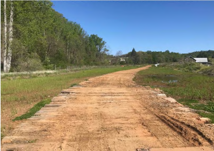
Figure 3: Stream S-E29 – Unnamed trib. to Teels Creek crossing looking downstream towards Teels Creek confluence. Incised stream banks covered in stabilization matting within ROW.
