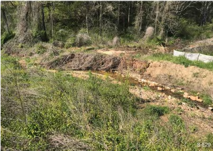
Figure 3: Stream S-E29 – Unnamed trib. to Teels Creek crossing looking downstream towards Teels Creek confluence. Incised stream banks covered in stabilization matting within ROW.
