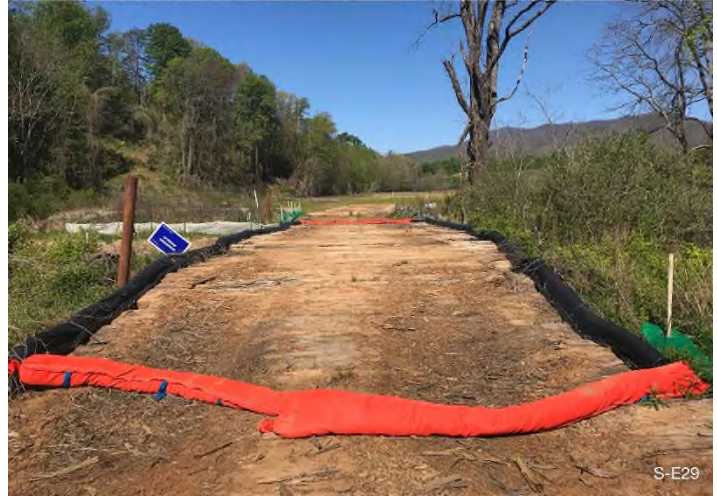
Figure 4: STA 13678+00 – Recent P1 repair along Teels Creek (S-E28). Note incised stream banks caused by stream meandering along inside bends.
