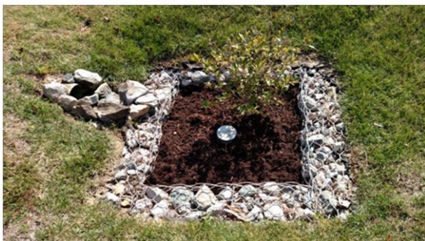
Figure 7.10. Manufactured urban stormwater BMP (Photo: Timmons Group)
