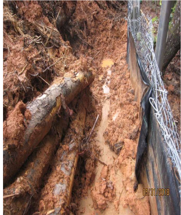
Sediment located on north side of SF
