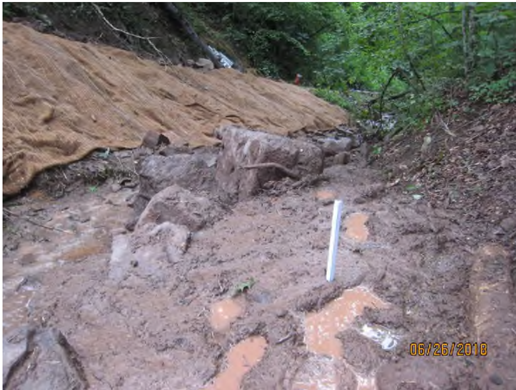
Photo 1: Sedimentation within "Stream 39" ~25' downstream of LOD
