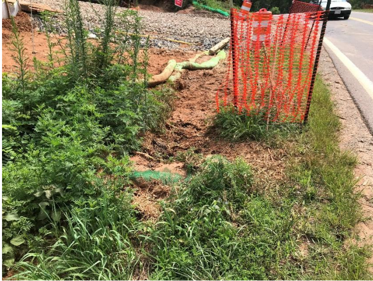
Compost filter socks check dams in roadside full of sediment
