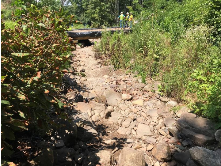
Channel downstream of crossing.
