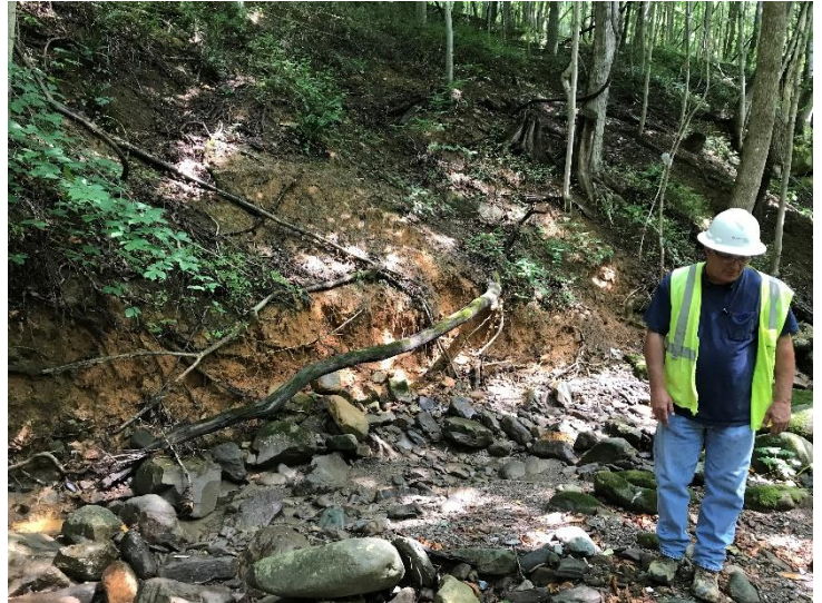
Existing eroding streambank upstream of creek crossing.
