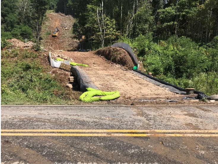
Doe Creek bridge crossing, E&S controls in good repair.
