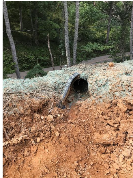
Fig. Near station 11776+80 slope drain observed lacked inlet protection
