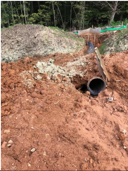
Fig. 3 Near station 11529+00 water bar observed required maintenance
