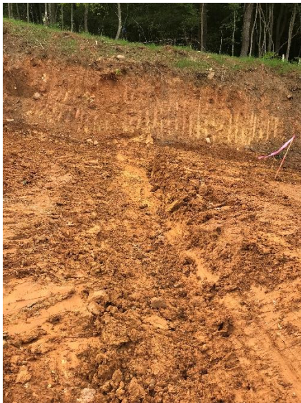
Fig. 3 Near station 11529+00 water bar observed required maintenance
