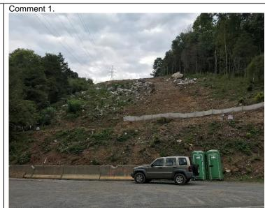
E&S controls in good condition on north side of Sinking Creek.
