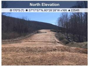
Figure 4: Above designated stream crossing S-NN12, ECD's and stabilization in place.
