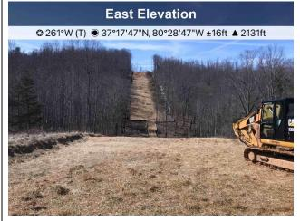
Figure 2: Near St11310+00 the area has recently been re stabilized with mulch.
