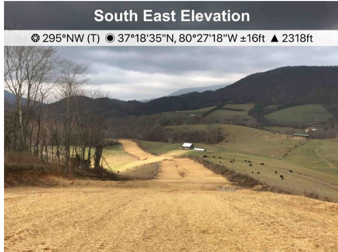
Fig. 1 Near MP 215.7 area has had stabilization applied.
