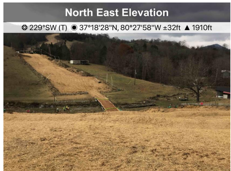
Fig. 4 Above designated stream S-KL43, ECD's in place and stabilization has been applied.
