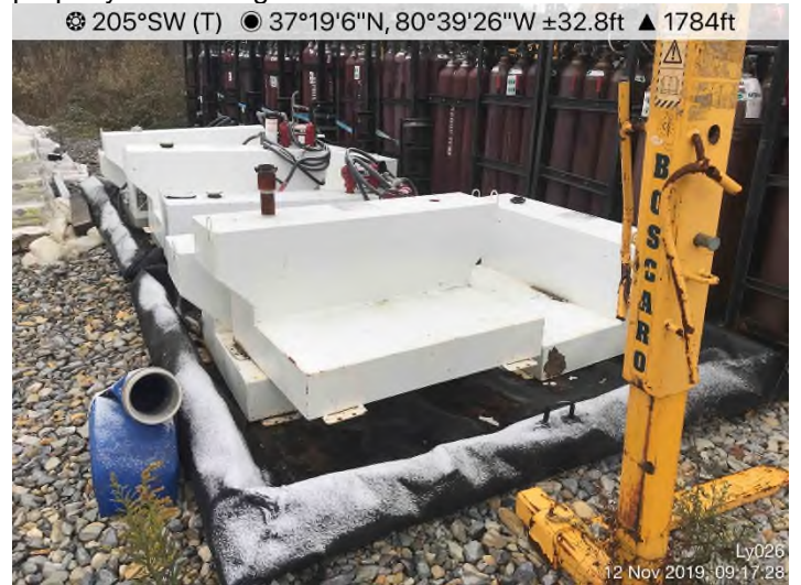
Fig. 4: Laydown Yard 028 – Secondary containment placed under equipment storage to contain potential leaks.
