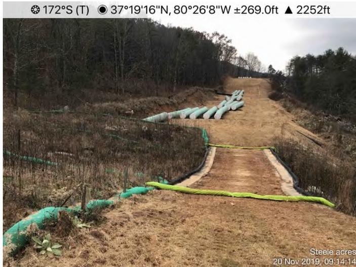
Fig. 2: **STA 11448+93** – Controls in place and functioning properly along Stream S-OO14. Area adequately stabilized with straw.
