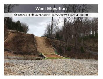
Fig. 2 Designated stream S-006, area near crossing is stabilized and ECD's are in place and functioning.
