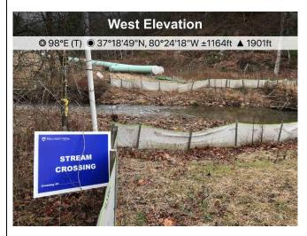
• Fig. 3 Designated stream S-RR13, area near crossing is stabilized and ECD's are in place and functioning.
