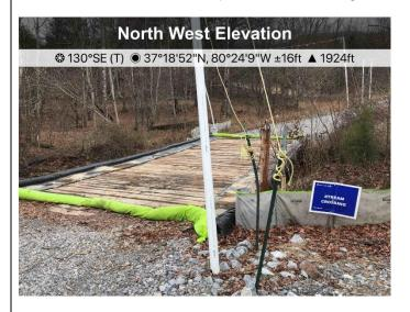
Fig. 4 Designated stream S-RR14, area near crossing is stabilized and ECD's are in place and functioning.
