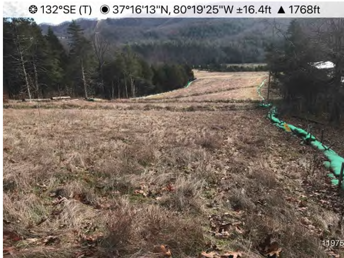
Fig. 7: STA 11975+00 – Looking south towards offsite karst feature. Controls in place. Area stabilized with vegetative cover. No erosion evident.
