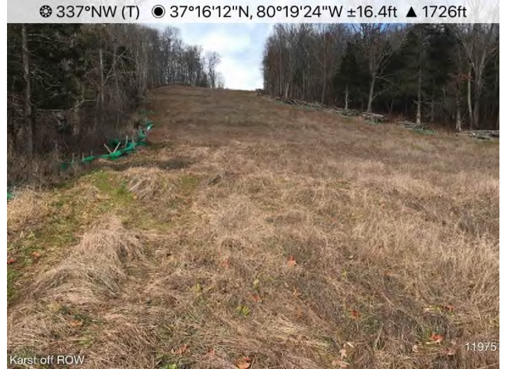
Fig. 8: STA 11975+00 – Controls in place. Area stabilized with vegetative cover. No erosion evident.
