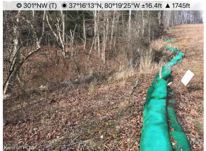
Fig. 8: STA 11975+00 – Controls in place. Area stabilized with vegetative cover. No erosion evident.
