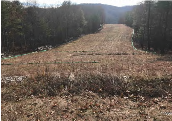
Fig. 3: STA 11956+00 – Controls in place and functioning. Area stabilized with vegetative cover.
