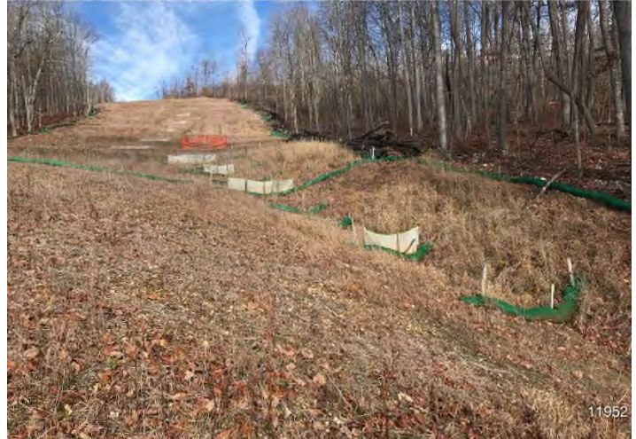
Fig. 4: STA 11974+00 – Controls in place and functioning. Area stabilized with vegetative cover. No erosion evident.
