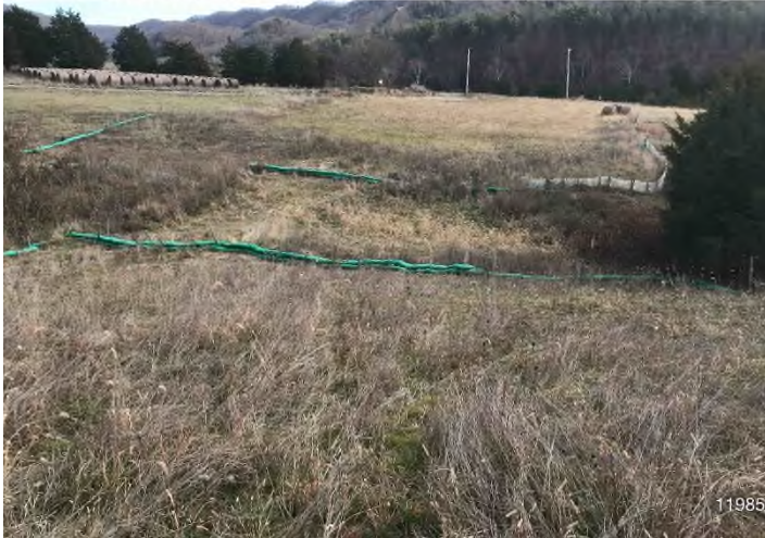
Fig. 15: STA 12004+00 – Controls in place and functioning. Area stabilized.
