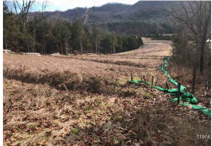
Fig. 4: STA 11974+00 – Controls in place and functioning. Area stabilized with vegetative cover. No erosion evident.
