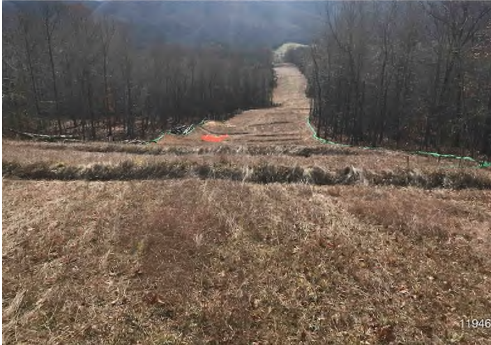
Fig. 3: STA 11956+00 – Controls in place and functioning. Area stabilized with vegetative cover.
