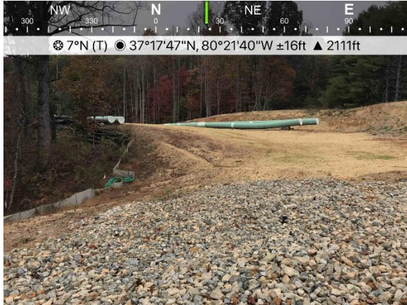
Fig. 1 ATWS 1487 has been stabilized and ECD's are in place and functioning.
