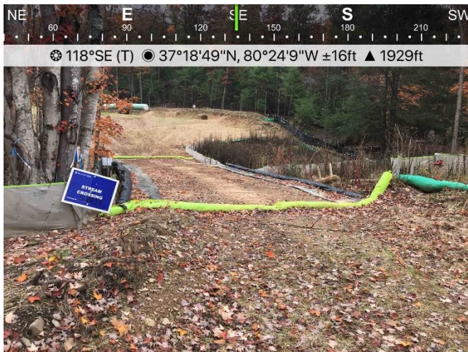
Fig. 3 Designated stream S-RR14, ECD's are in place and functioning.
