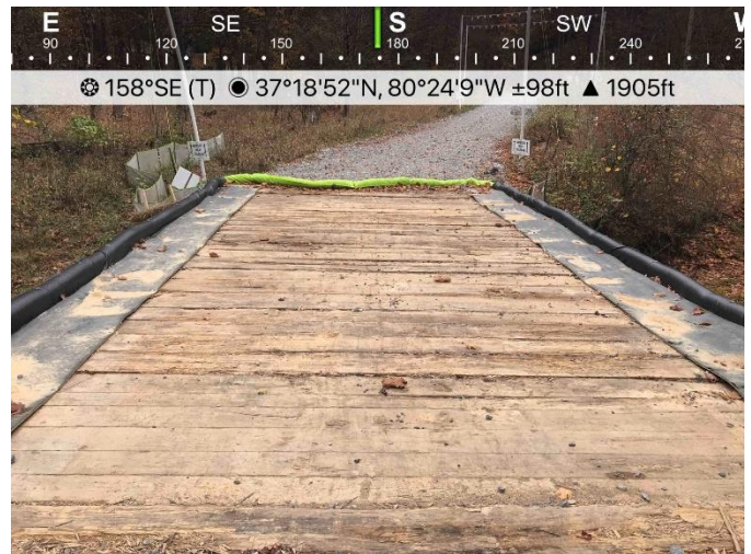
Fig. 4 ATWS 1057 & designated stream S-RR13 ECD's are in place and functioning.
