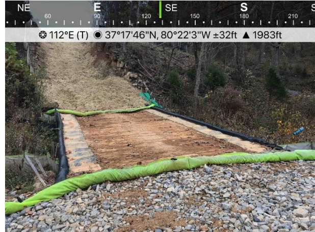
Fig. 2 Designated stream S-IJ 52, ECD's in place and functioning.
