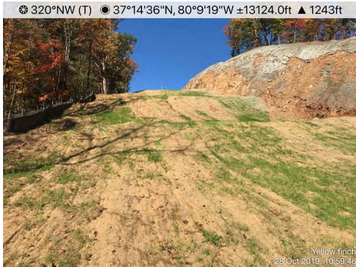
Fig. 3: STA 12541+00 – Stockpile slipping onto ROW. Item identified by MVP on 10/20/2019. Repair extended due to wet ROW conditions. Controls in place and functioning at the time of inspection.
