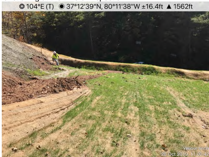
Fig. 3: STA 12541+00 – Stockpile slipping onto ROW. Item identified by MVP on 10/20/2019. Repair extended due to wet ROW conditions. Controls in place and functioning at the time of inspection.
