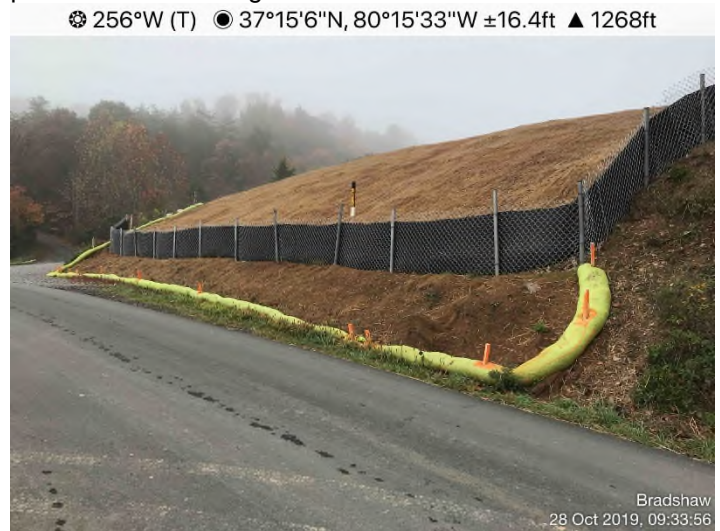
Fig. 4: Stream S-C21 – Looking downstream at Bradshaw Creek crossing. No evidence of sediment discharge from ROW. Controls in place and functioning.
