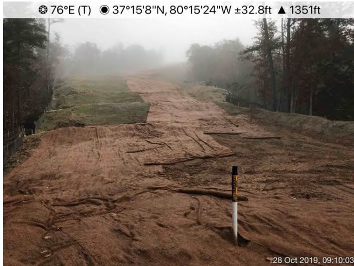
Fig. 3: Stream S-C21 – Looking upstream at Bradshaw Creek crossing towards Bradshaw Road. No evidence of sediment discharge from ROW. Controls in place and functioning.
