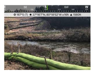
Fig. 4 Near MP225.9 area is stabilized and ECD's are in place and functioning.
