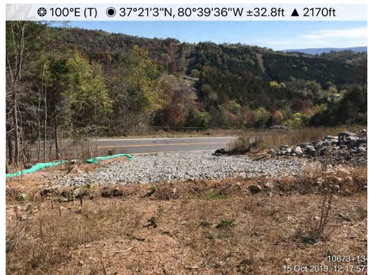
Fig. 4: STA 10673+13 – Controls in place and maintained properly at Big Stoney Creek Road.
