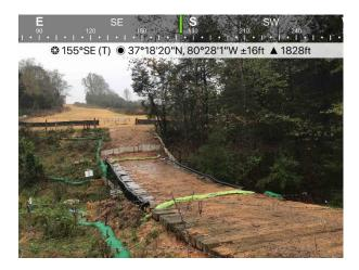
Fig. 2 Near MP 214.4 stabilization has been applied and ECD's are in place and functioning.
