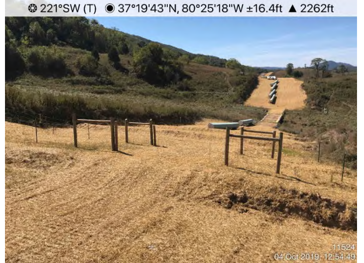
Fig. 4: STA 11524+00 – Controls in place. Area stabilized.
