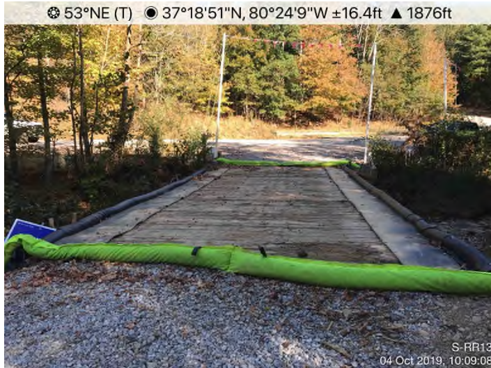
Fig. 3: Stream S-002 – Sinking Creek crossing, downstream view. Controls in place and functioning properly.
