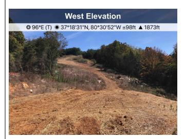
Fig. 3 At St11816+00 stabilization has been applied with permanent style water bars with level spreaders.
