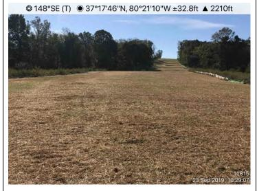
Fig. 4: **STA 11890+00** – Controls in place. Area stabilized with seed and straw.
