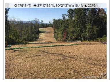
Fig. 2: **STA** 11815+00 – Controls in place. Area stabilized with seed and straw.
