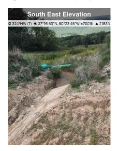
Fig. 2 Near ST11354+00 area has been stabilized with seed and mulch
