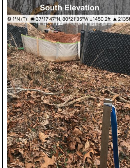
Fig. 4 St#11764 no sediment observed off the ROW
