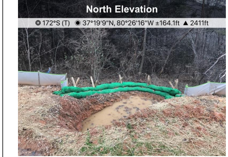
Fig. 2 At St#11459+00 no sediment observed off the ROW
