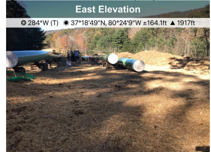
Fig. 4 St#11600-11613 has been adequately mulched.
