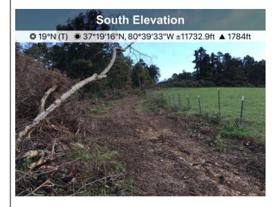
Description: At designated stream G-32 ECD's have been repaired and escaped sediment has been remvoed.
