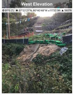
Description: At St#11064+84 slope lacks stabilization.
