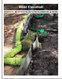
Description: At designated stream SM N 21 ECD's have been repaired and escaped sediment has been removed. **West Elevation**
