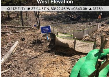
Description: At designated stream S- MN 22 ECD's have been repaired and escaped sediment has been removed.
