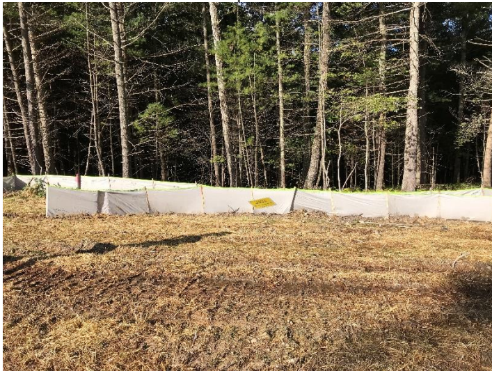
Fig. 3 MP 226.37 karsts feature protected
