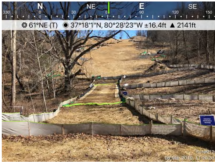
Fig. 3: S-NN12 – Area adequately stabilized. Controls in place.
