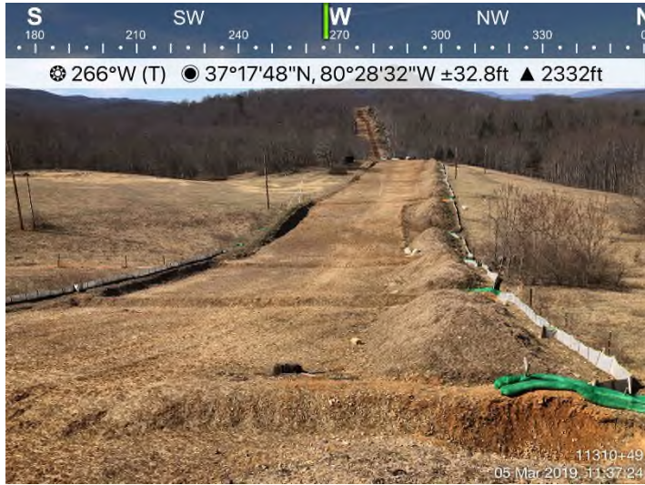
Fig. 7: STA 11345+68 – Area adequately stabilized. Controls in place.
