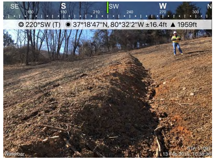
Fig. 4: STA 11097 – Waterbar does not meet slope requirements.
